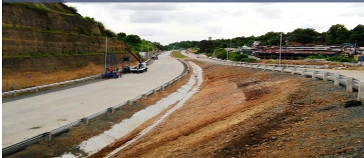
Daang Hari-SLEX Link Road Project
