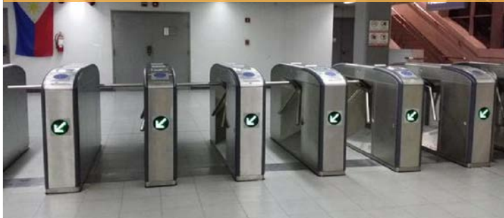
Automatic Fare Collection System
