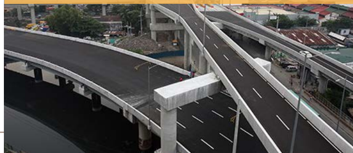
NAIA Expressway Project (Phase II)
